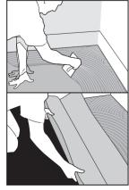
3. Apply **LVT 920 Tackifier** to the sub-floor using a roller, trowel or brush.
