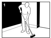
The sub-floor must be level sound, dry and free from dust, grease and other contaminants.
