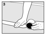
Tape all joins with a suitable single sided moisture proof tape<sup>†</sup> and press firmly into place.
